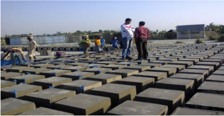
Manufacturing of CC Block and Laying of Blocks
