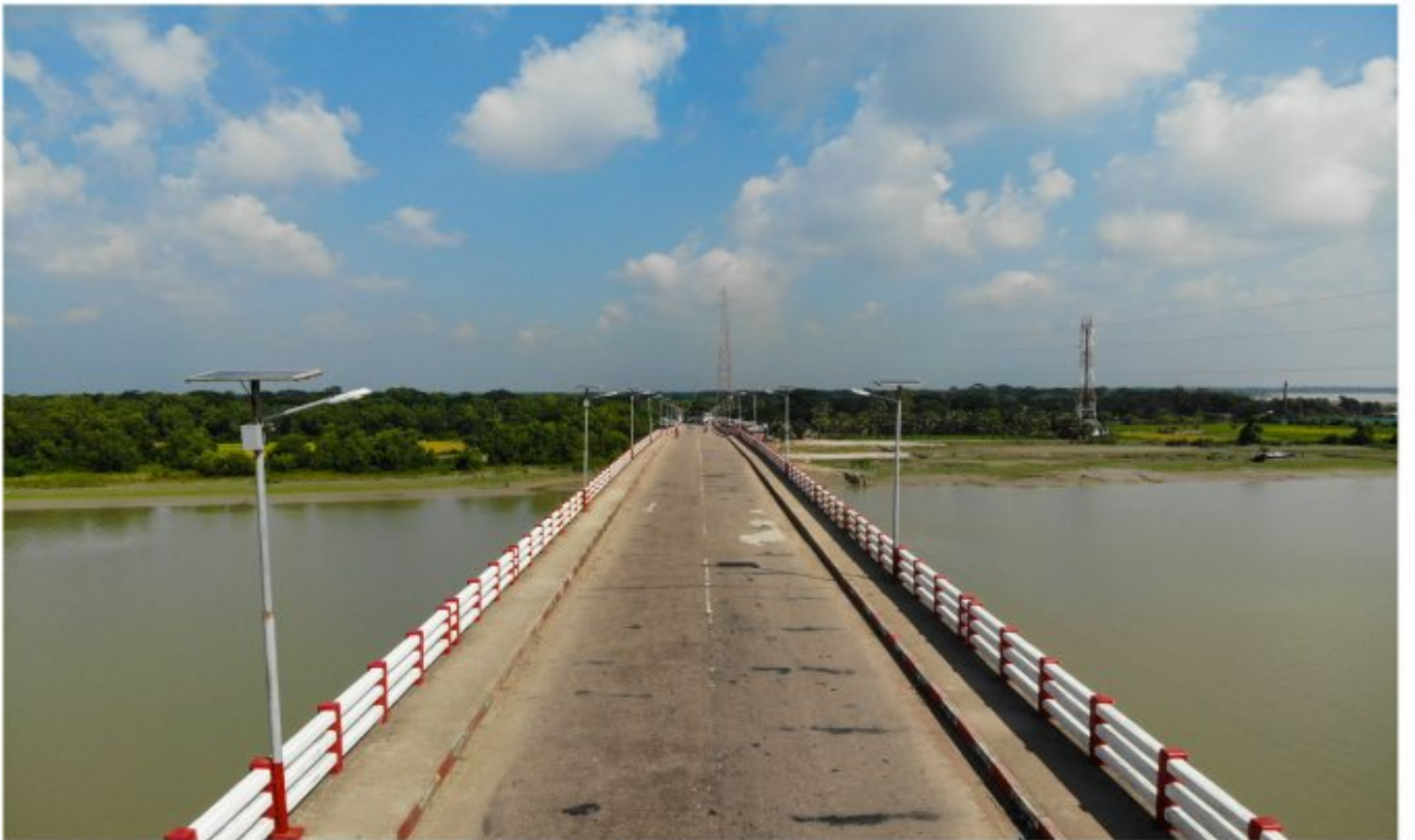
Construction of 482.375m (2X42.68m+8x48.80m) Long P.C Girder Bridge (Hazipur Bridge) Shahid Shiekh Jamal Bridge at 61st km of Patuakhali-Kuakata Road under Patuakhali Road Division During the year 2009-2010. Procuring Entity: Roads and Highways Department (RHD) Contract Amount: BDT 52,41,11,211.74. USD 7.00 Million Completion Date: 07/03/2012 to 22/06/2017.
