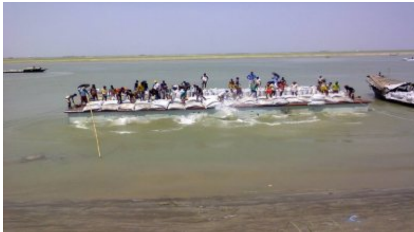
Dumping of Geo – Bag & Synthetic Bags
