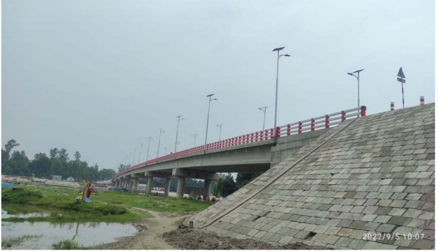
Construction of 294m long PSC Girder Bridge Over Fulzhury River on Barahar UP Office-Tetulia Hat road, Ullapara, Sirajgonj
